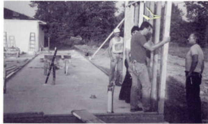
Erection of first stud wall for sanctuary.
