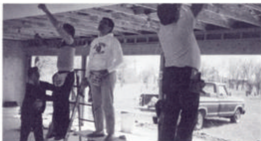
Shelter construction began in spring of 1986.
