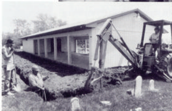
Digging footer for new sanctuary.
